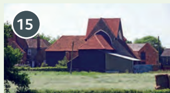
15 Latton Priory (Listed Building)
